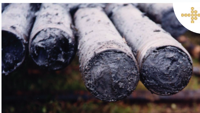
Production tubing totally blocked by crude heavy deposits.
